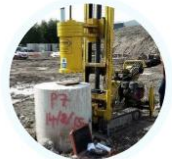
Pile Load Testing
