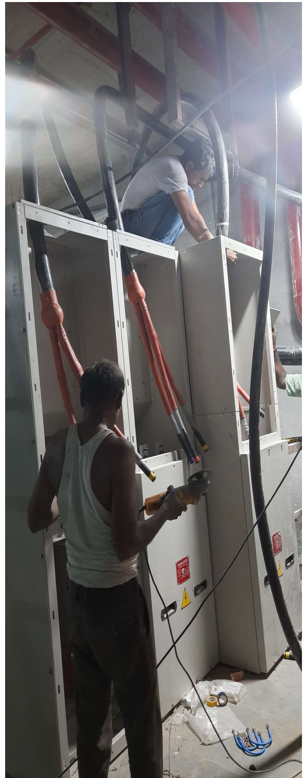
Al-Jamea HT Panel Cable Termination
