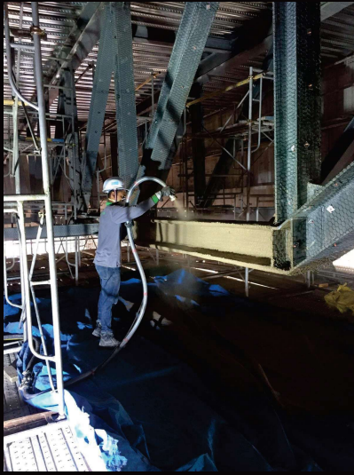
Structural Steel Protection using Vermiculite Spray
