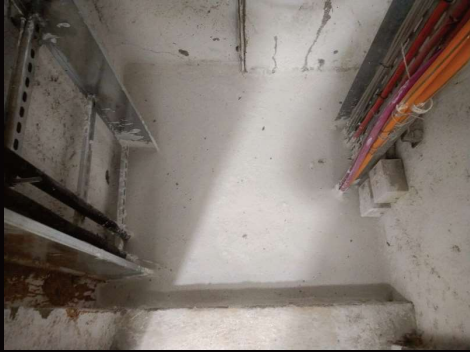
Firestopping for penetrations through floor
