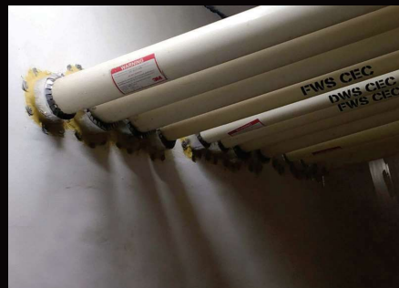
Fireproofing of Pipe Penetrations
